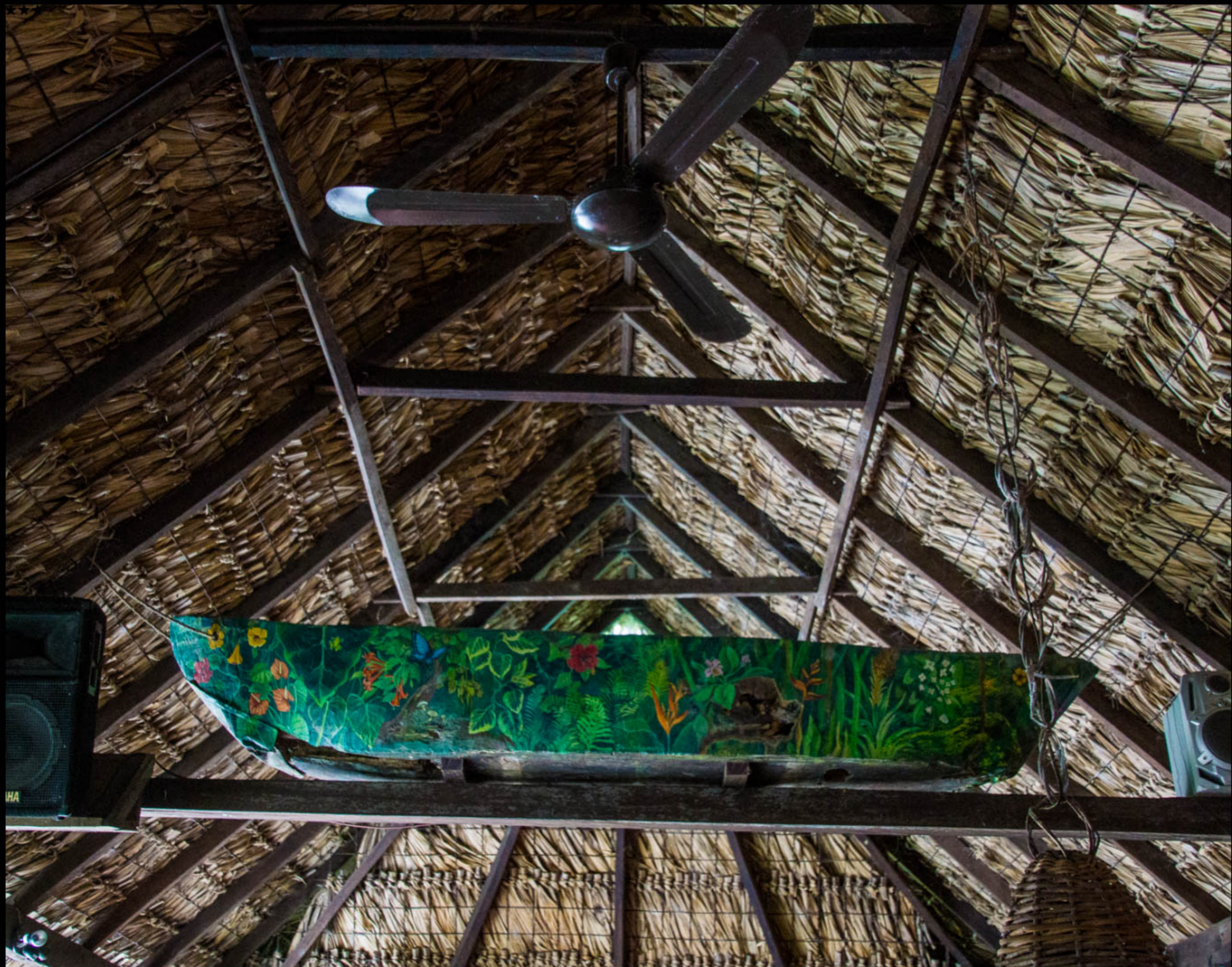
Roof of restaurant
