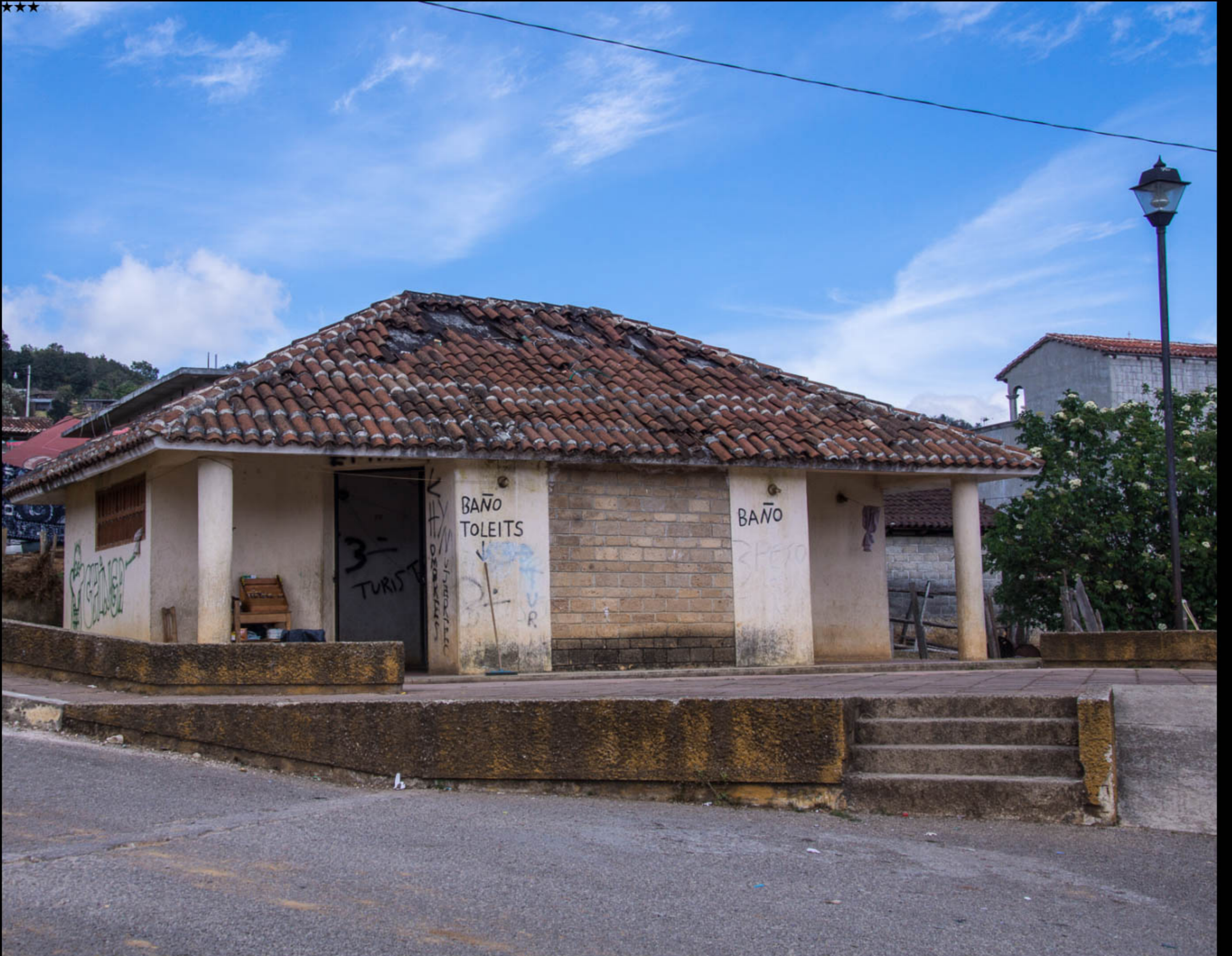
Public toilets in tourist parking lot
