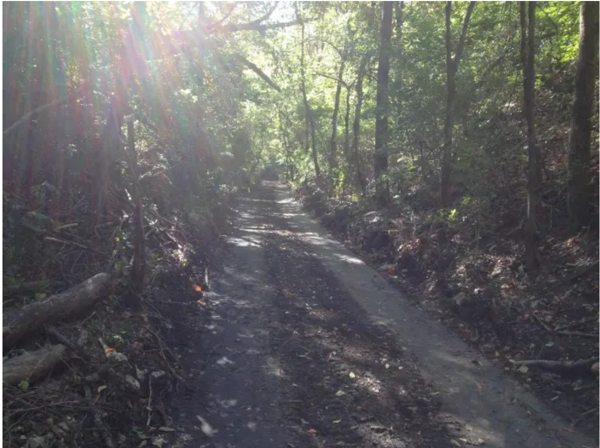
Original Road Bed being improved/new trail construction
