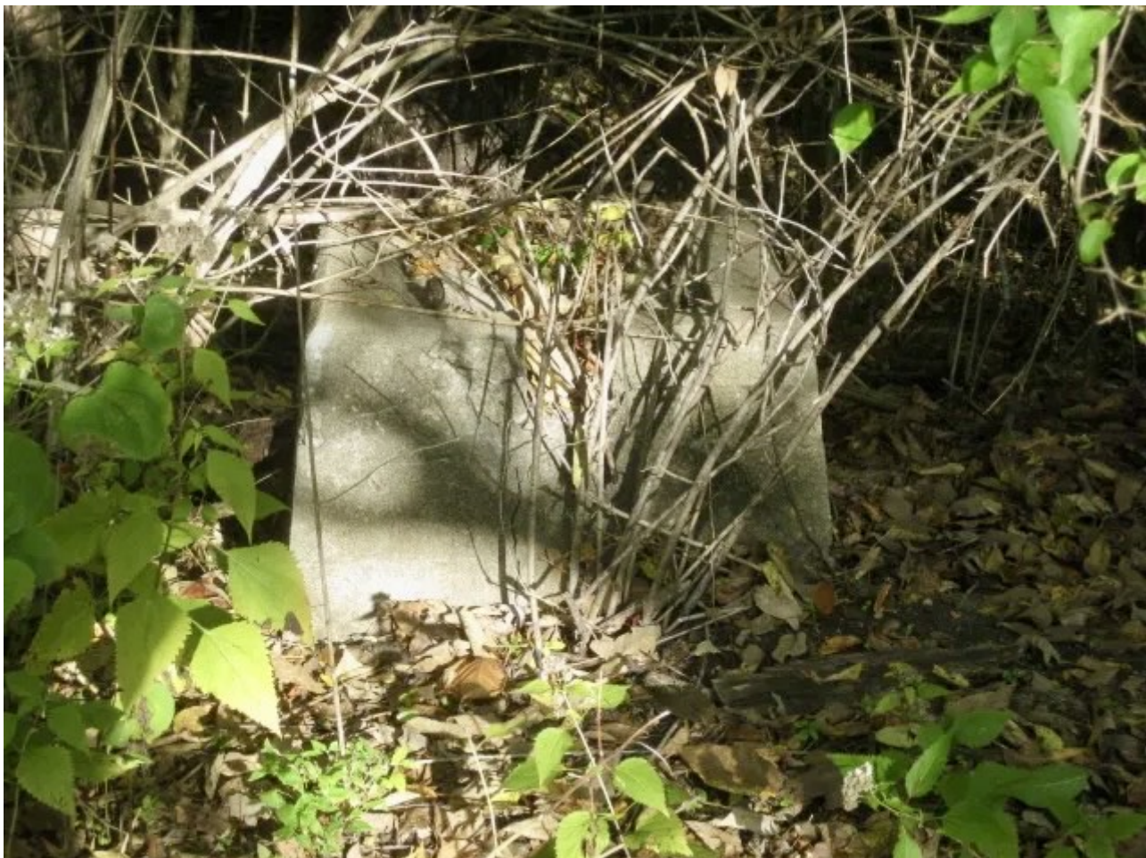
Concrete Power Pole footing Martha Lafite Thompson
