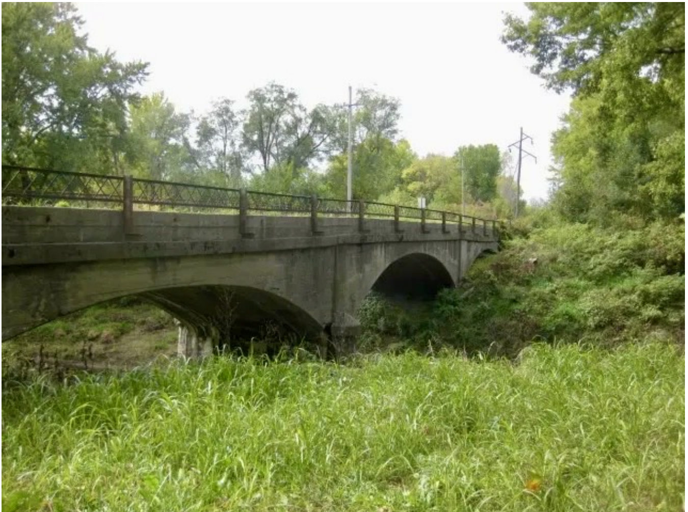
Main Street Bridge looking South, third arch partially obscured Mosby, MO
