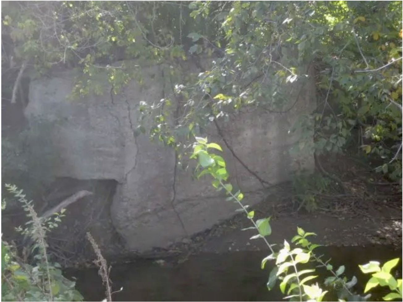
Bridge Abutment along Waukomis Dr
