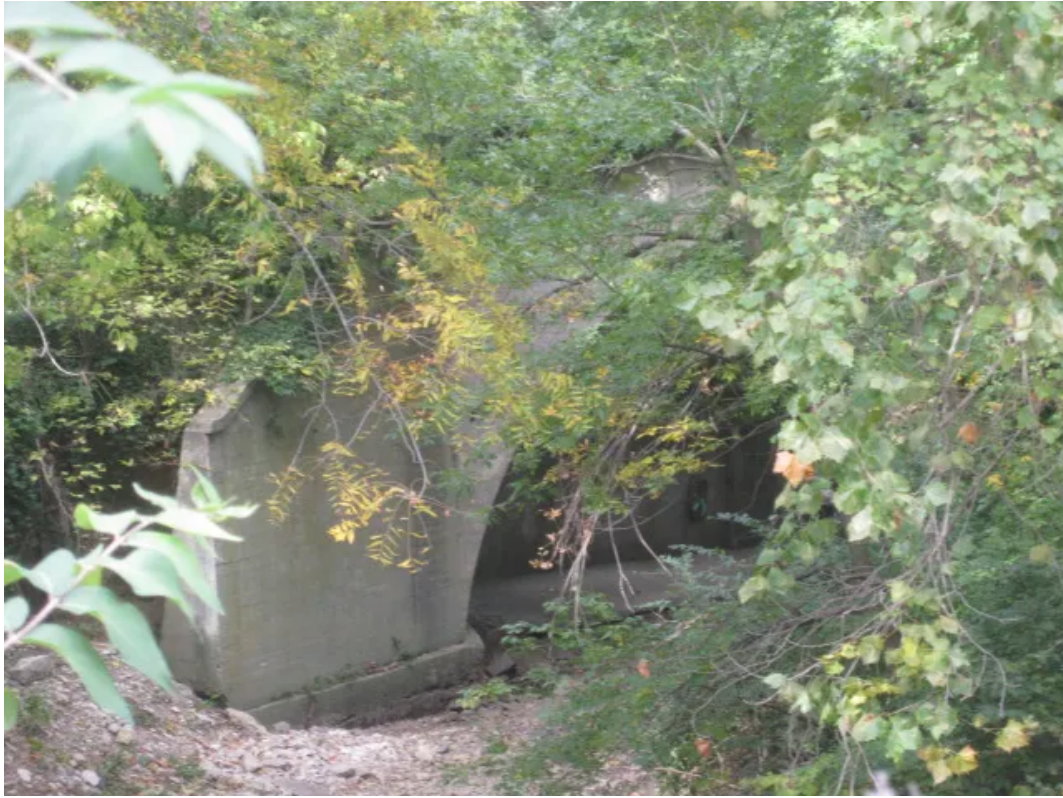
Single Arch Bridge
