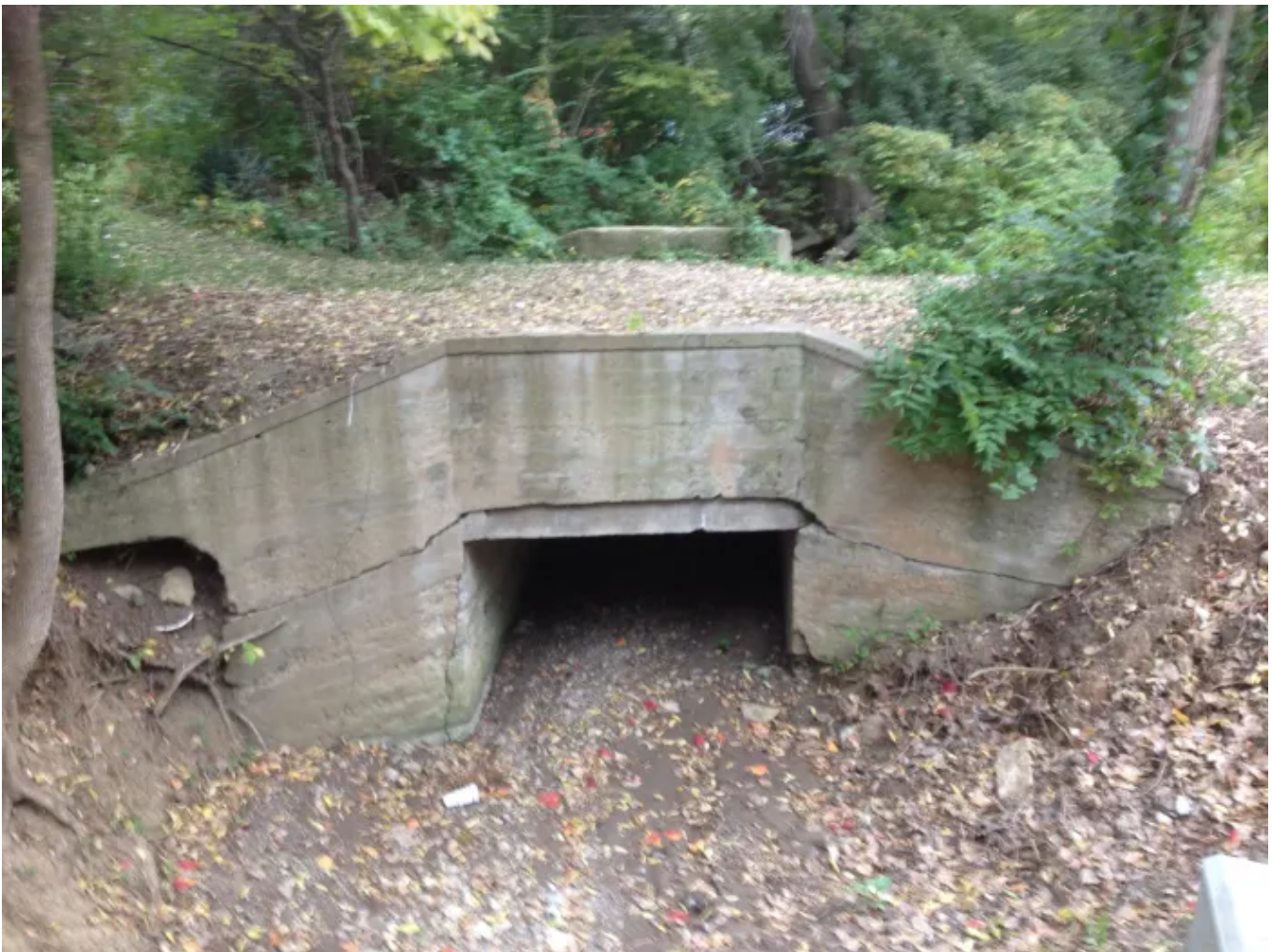
Concrete Box Culvert beside Waukomis Rd .1 mile South of 68th
