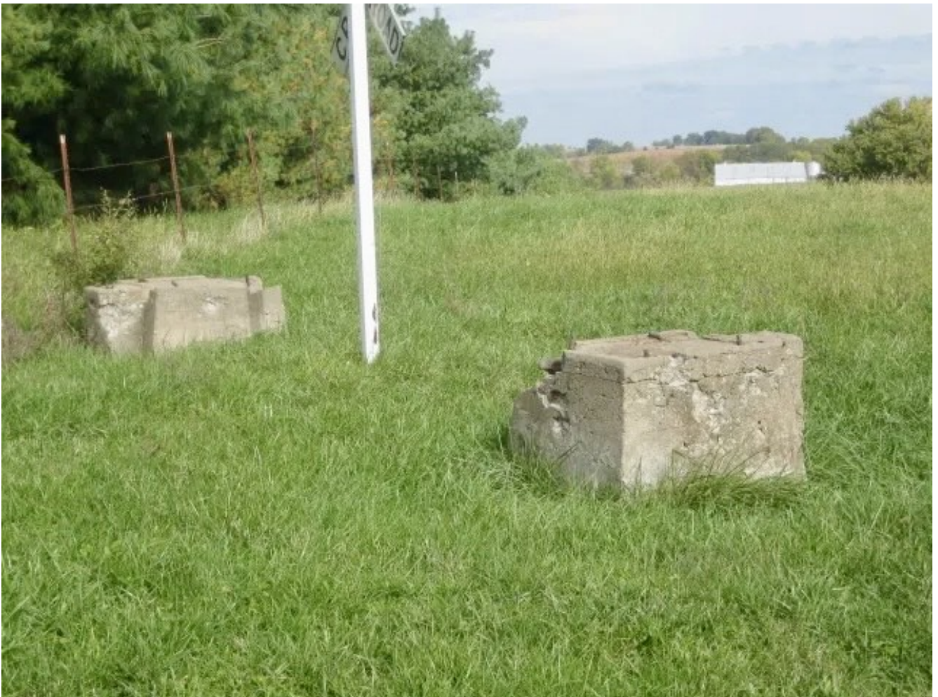
Opposed concrete power pole footings, Hwy H East of Liberty
