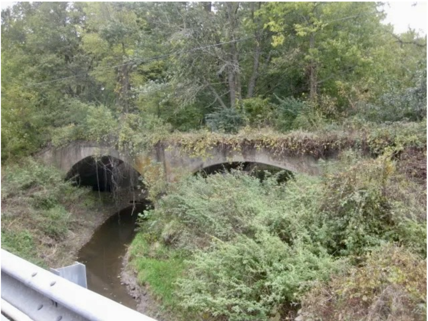
Double Arch Prathersville Bridge crossing Williams Creek
