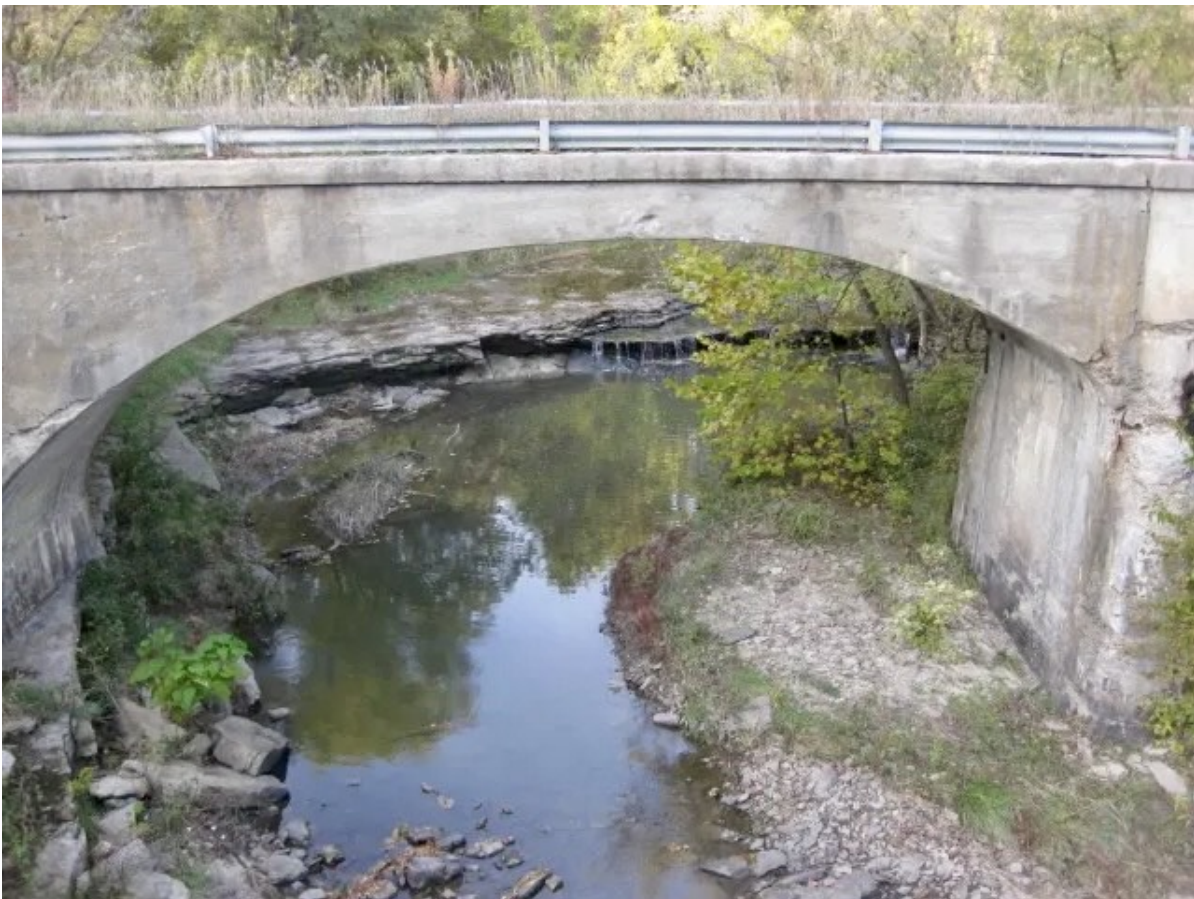
South Arch of Todd Creek bridge
