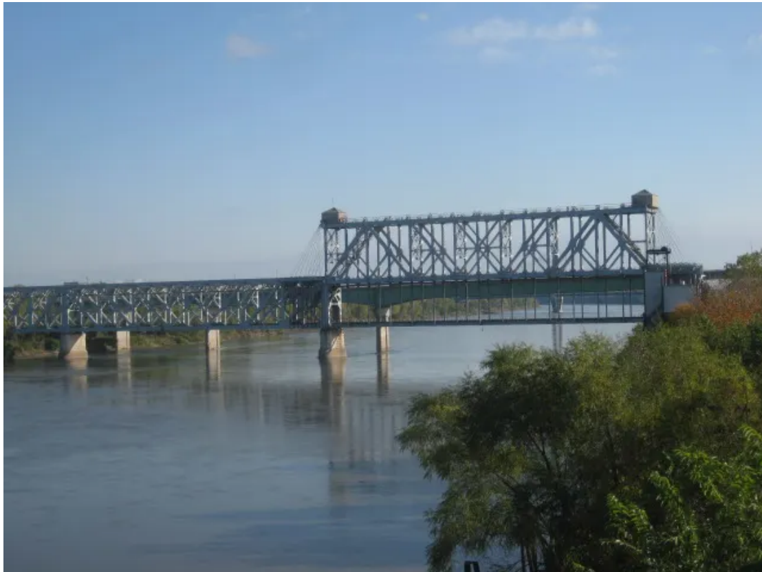
ASB Bridge looking East
