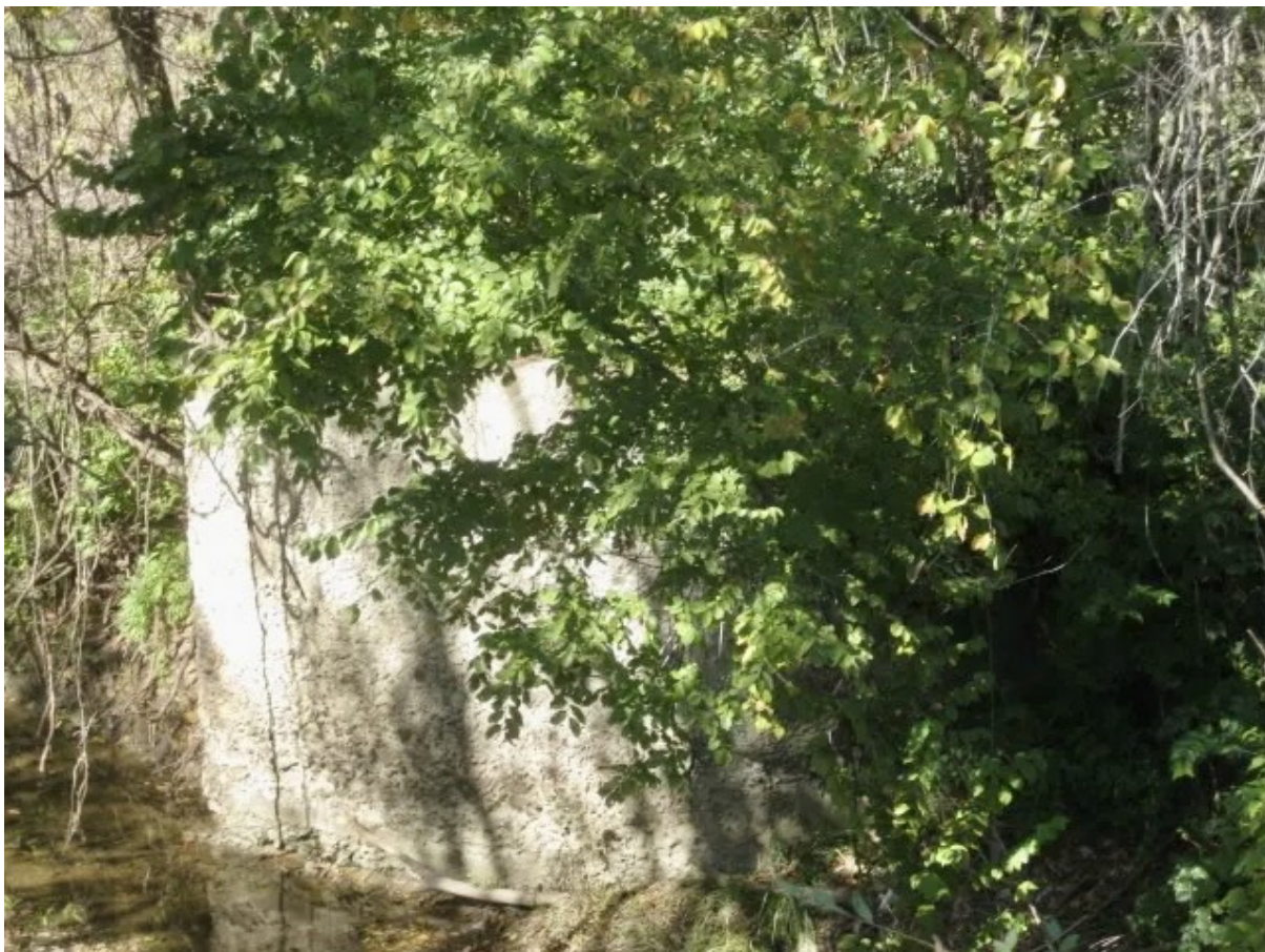
Bridge Abutment peeking out of bushes
