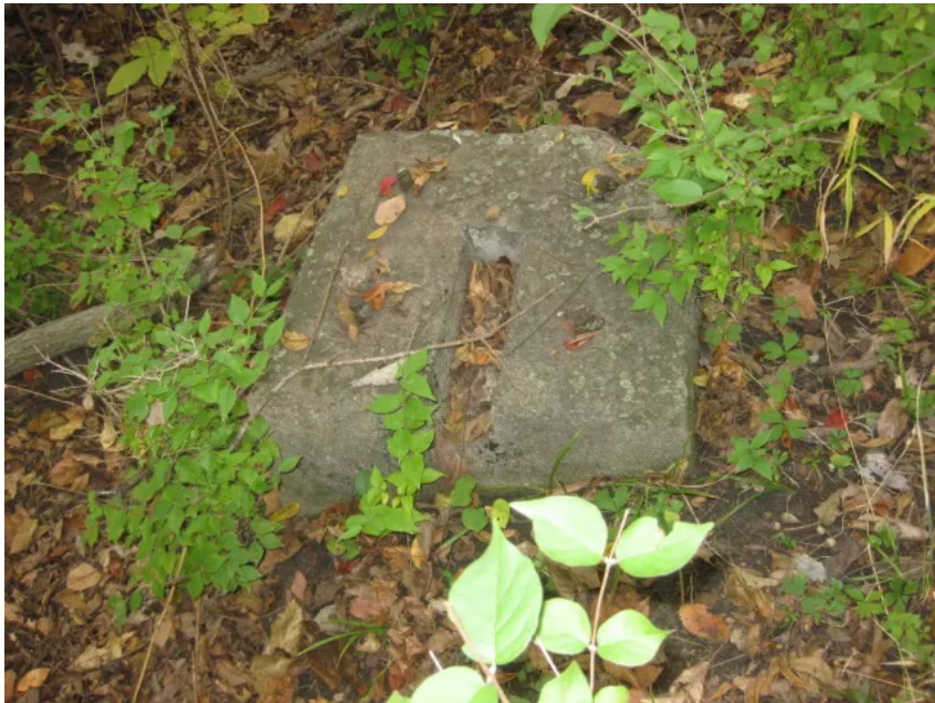
Concrete Pole footing
