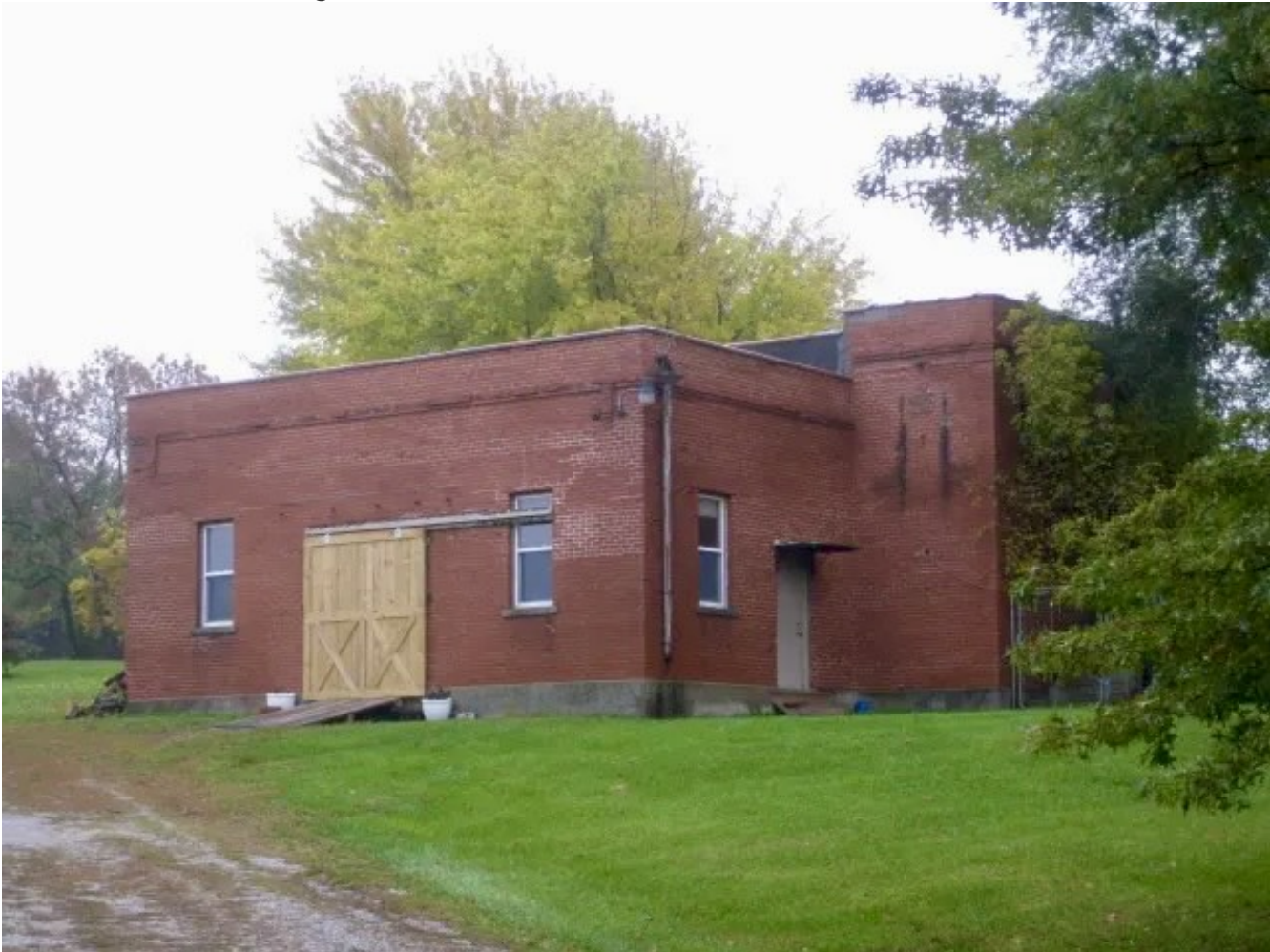
DC Power Generation Station
