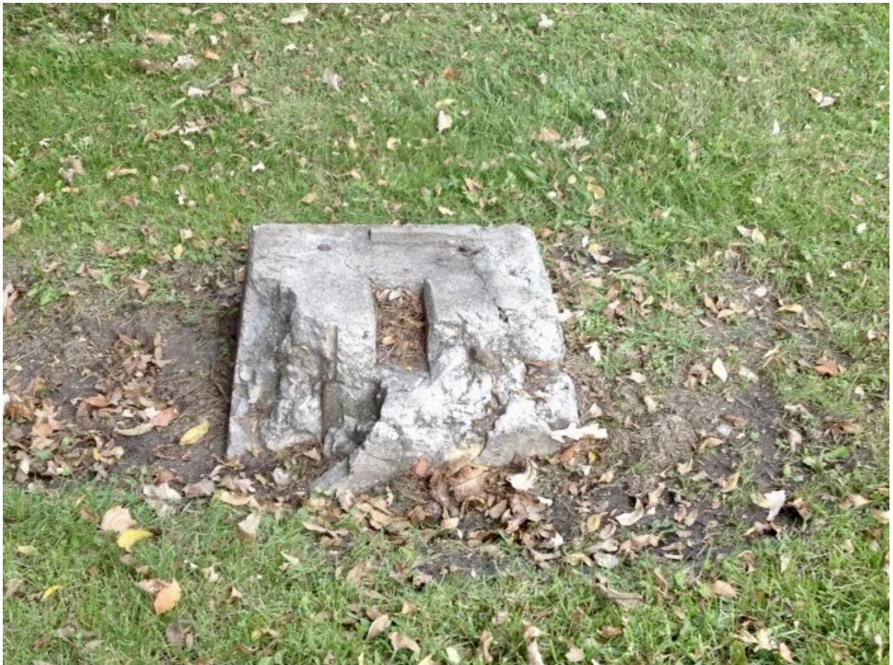
Power Pole footing along side Trail Westboro Canterbury Greenway
