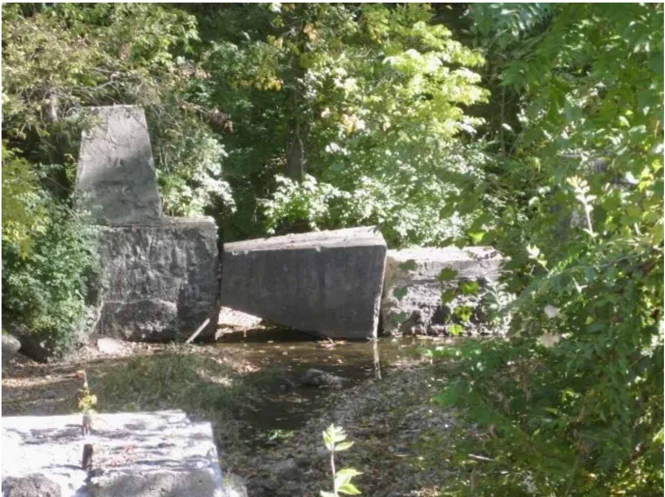
Avondale Trestle Footings in Rock Creek
