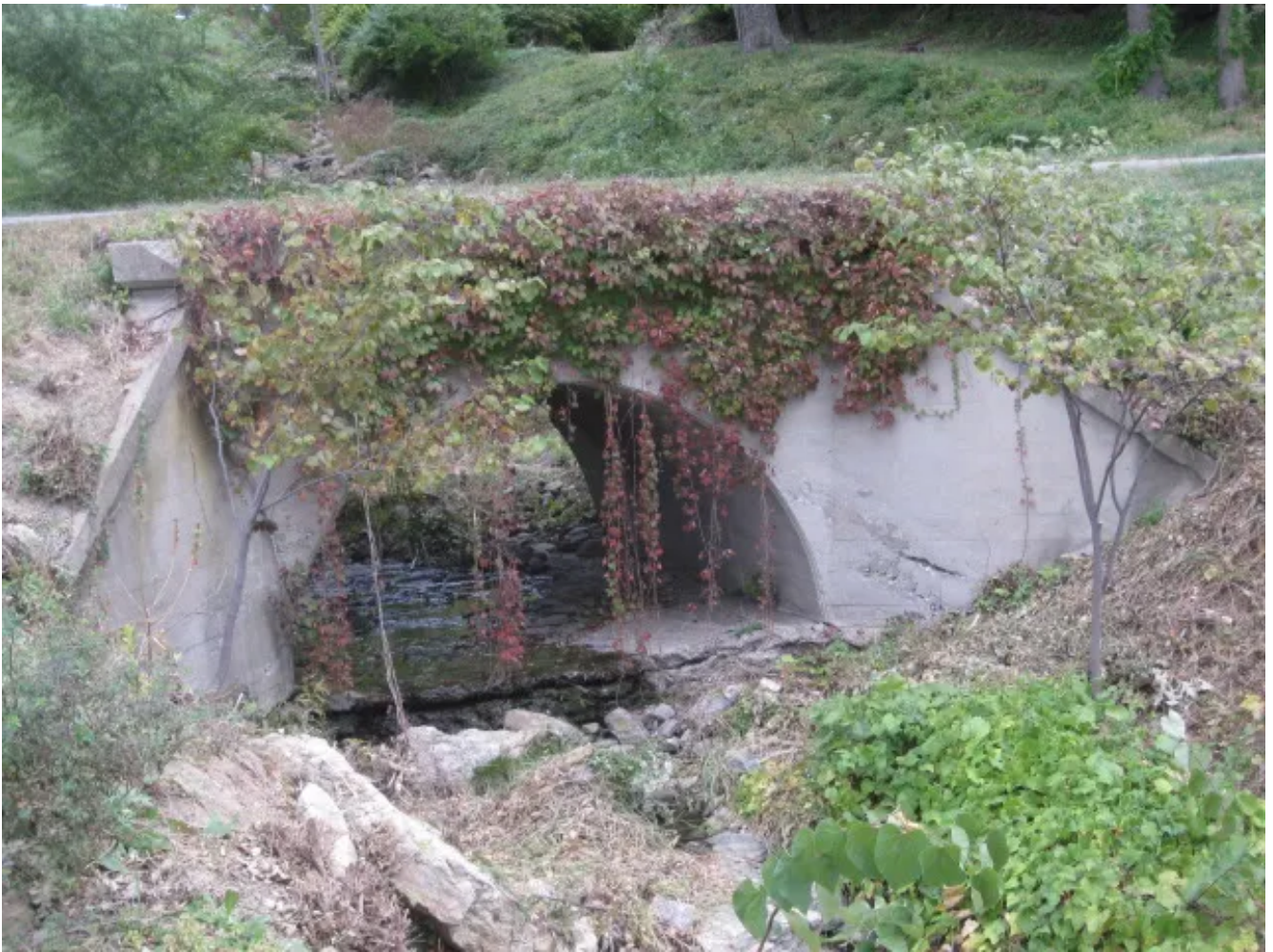
Single Arch Concrete Bridge HWY 9/NW Platte Rd Trail
