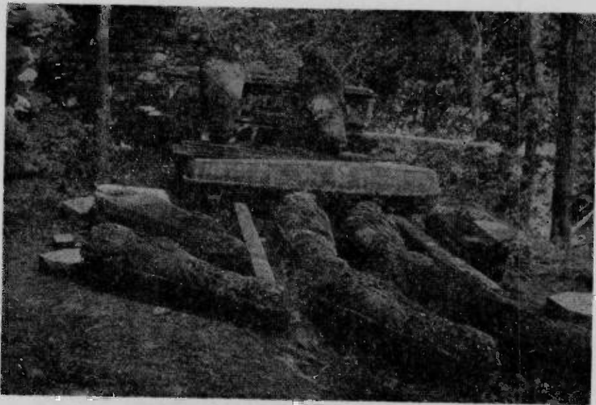
IRON COFFINS IN WHICH THE LAIRS ARE BURIED
